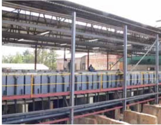
Sable copper electro-winning tankhouse
